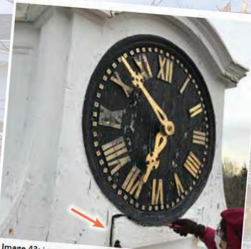
Image 43: Loose and deteriorated boards at the clock require repair and refastening.
