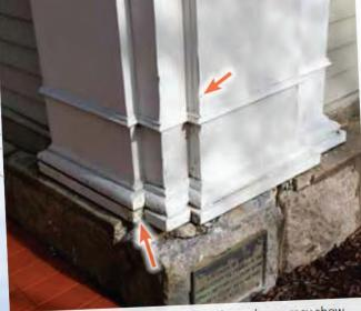
Image 07: Wood mouldings at the pilaster bases may show more wear due to snowbanks and splashing rainwater.
