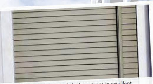
Image 01: In general, wood clapboards are in excellent condition, both tight and sound.
