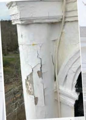
Image 39: Peeling paint on the columns require scraping, sanding, and new paint.
