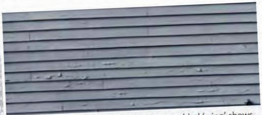
Image 02: One instance at the northeast gabled 'wing' shows peeling paint and visible joints.
