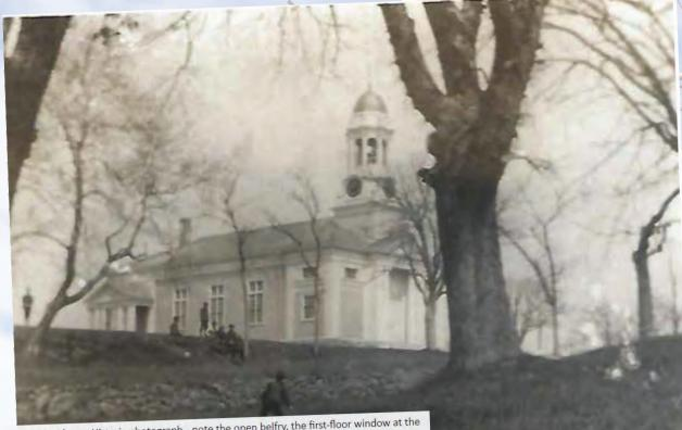
**Image Above:** Historic photograph - note the open belfry, the first-floor window at the front of the south elevation, and the chimney on the western roof slope.
