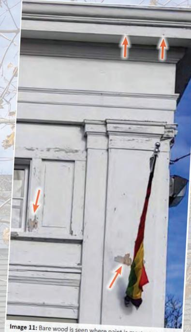
**Image 11:** Bare wood is seen where paint is most worn or peeled altogether. Small nail heads are visible throughout.
